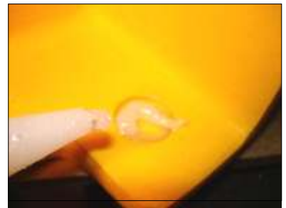
3. Apply silicone to the inside of the hole
